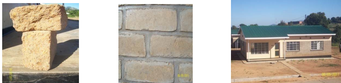
Figure 1: Example of Alternative Building Material and the Related Structures: Stabilised Soil-Cement Blocks for Mass Housing Projects in Malawi (Photos by EC Mpakati Gama, May 2011)
