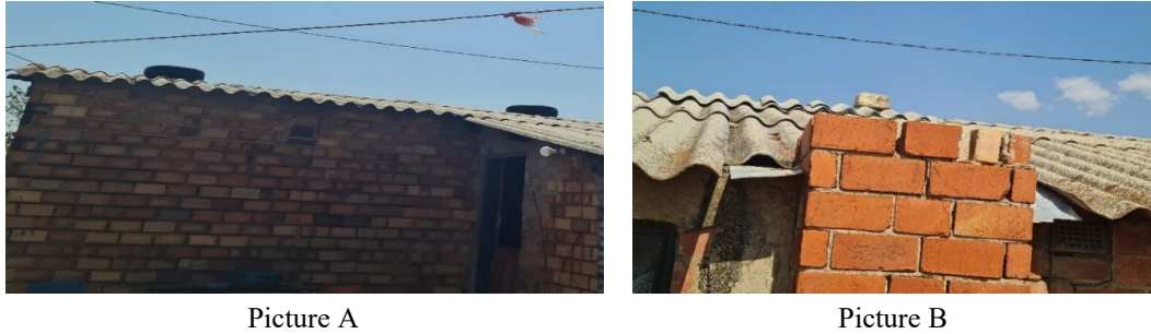
Figure 1: Pictures of an unsecured asbestos roof support against the wind
