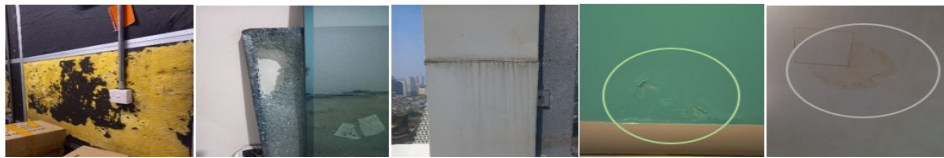
Figure 1: Insulation defects
