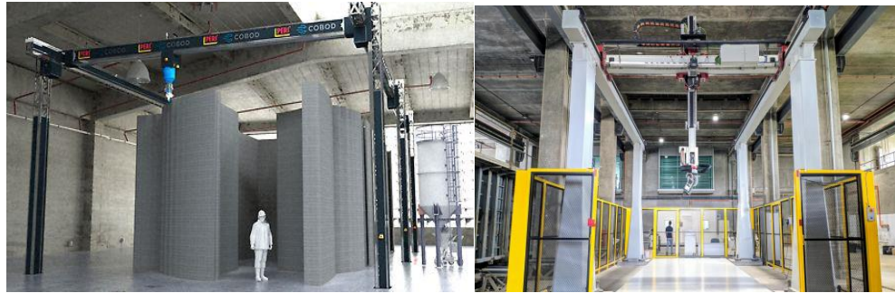
Figure 1: 3D Concrete Printing Applications in Building
