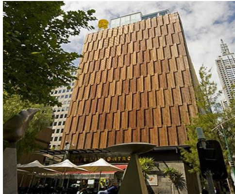
Figure 4: Council House, Melbourne
