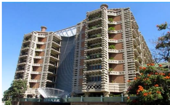
Figure 3: East Gate Center, Harare
